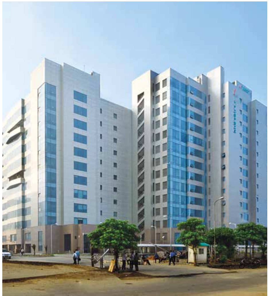
The word 'façade' means the complete envelope and there are permutation and combination of various materials, which could be considered for it.
